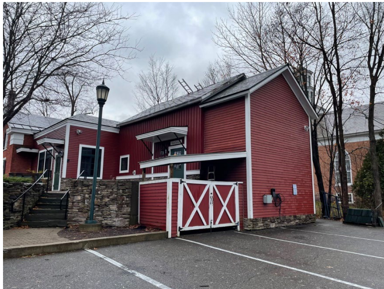
Photo: November 2024 2004-06 renovations included a new hipped roof "link" replacing original 1840 ell adding approx. 300 sq. ft. Barn is elevated and relocated. Renovated barn has new window and pedestrian door on east side; north gable end windows removed and two story stair tower added (2004-06 building project).
