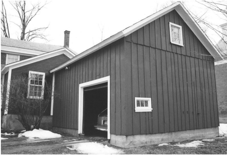
C.1840 Barn, attached to historic c.1840 ell. Wood board and batten siding described as replaced (1992). Poured concrete foundation. Overhead garage door within the original barn opening. View looking southwest. Williston Village Historic District, Boundary Addition. Entered on the National Register, October 1992. Photo 1991, credit Ann Cousins.
