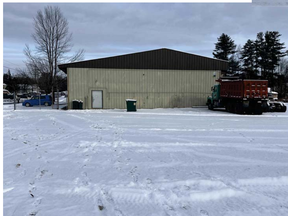
View of Southern face of existing building (side of Building Addition)
