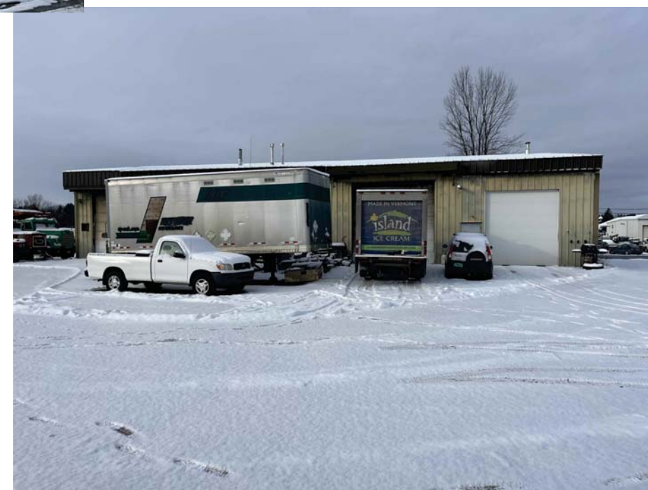
View of Eastern face of existing building
