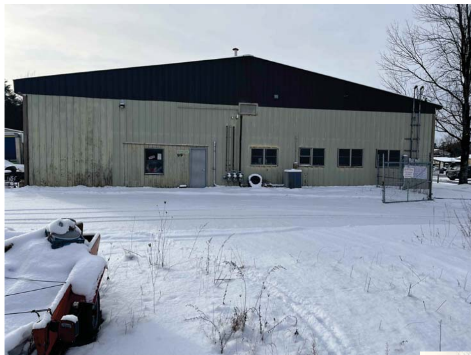
View of Northern face of existing building
