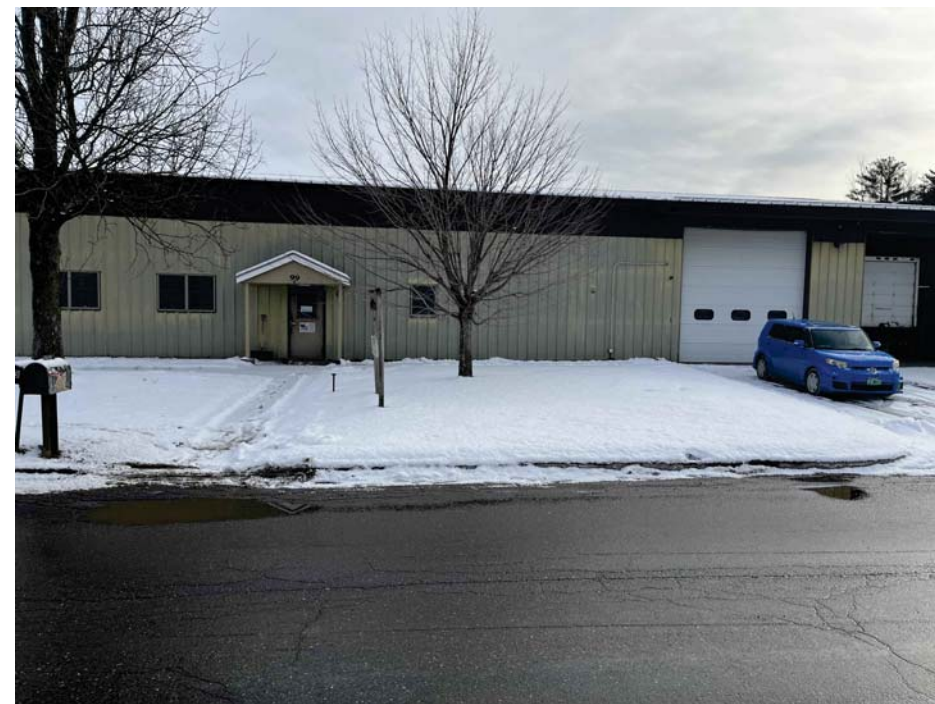
View of Western face of existing building from across Engineers Drive
