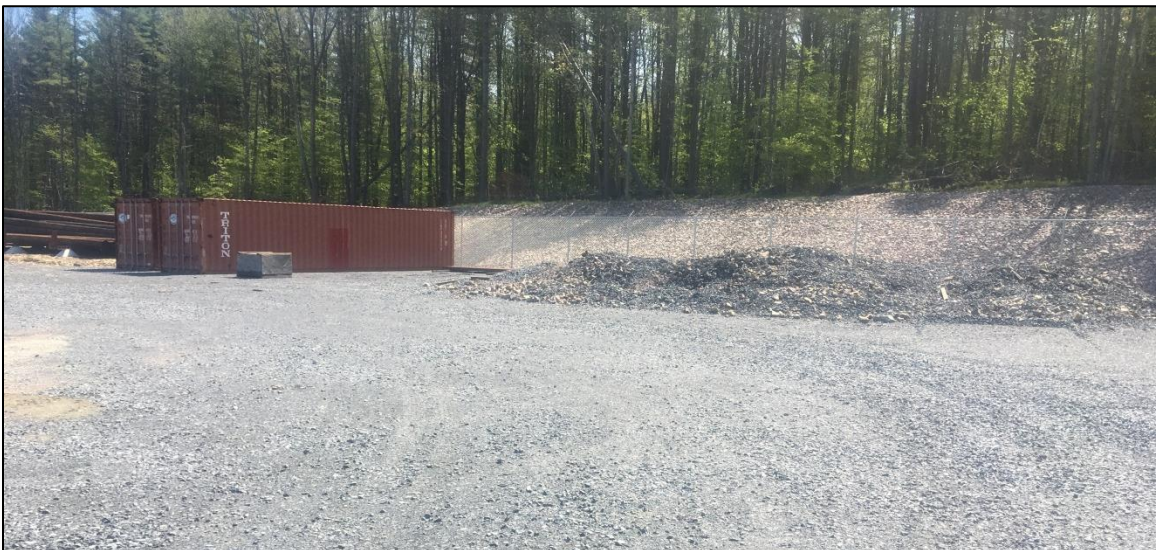
Photo 2: View of the location of the proposed building within the existing gravel storage yard.
