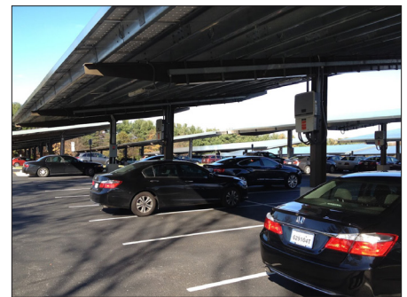
Illustration Solar Canopy over mid-BLOCK Parking
