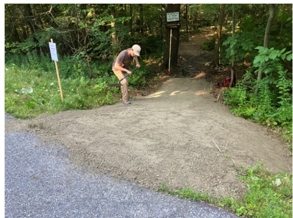
2 FotW working on the trail at South Road
