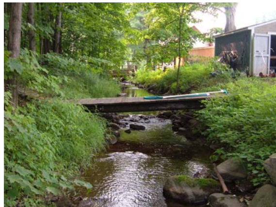
Figure 17. Corridor encroachment in T1.05-A
