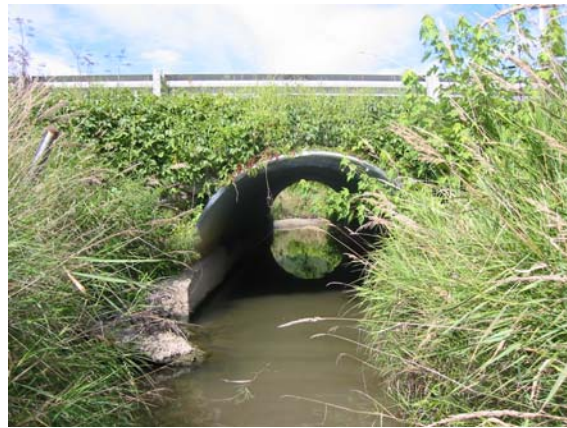
Figure 7. Culvert beneath Route 2A
